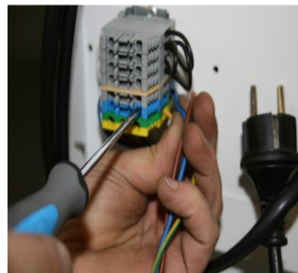
5 Connect power and remote humidostat wires.
