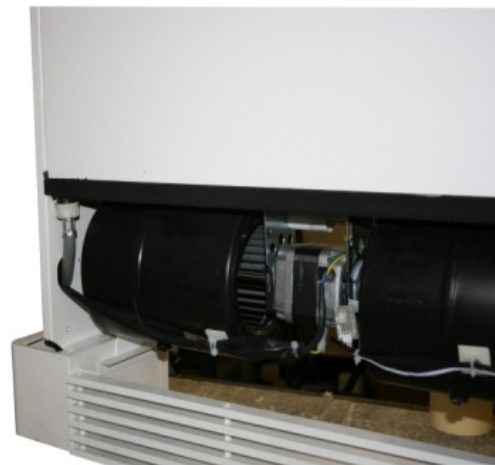
5 Connect power and remote humidostat wires.
